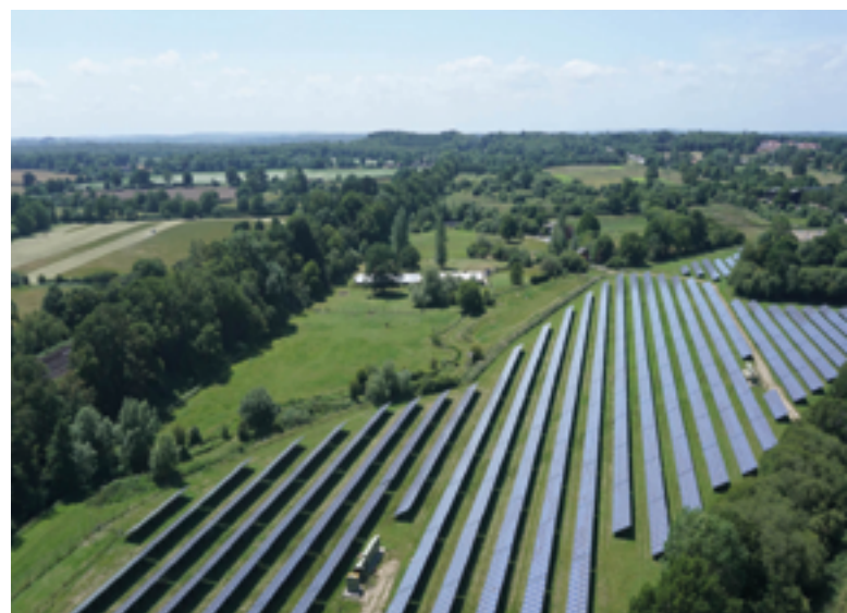
Oakfield Solar, Hampshire, UK, operated by DRD since 2020
